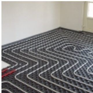
Henco Floor heating of plastic multilayer tube
